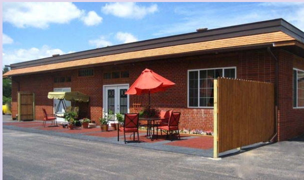
5—Neil Bretl N5620 Highway H, Antigo (Former River Grove School)
